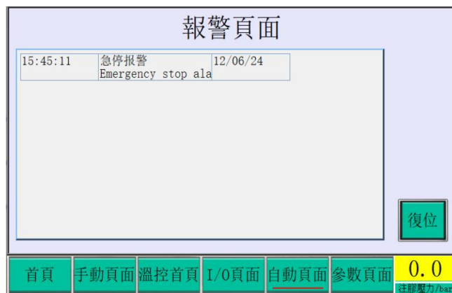
Figure 12: Emergency Stop Failure
